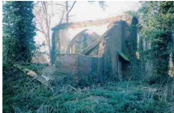
Ruins of Old St. Nicholas Church, Kelvedon Hatch, Essex County. (Photo Courtesy Kelvedon Hatch History)
